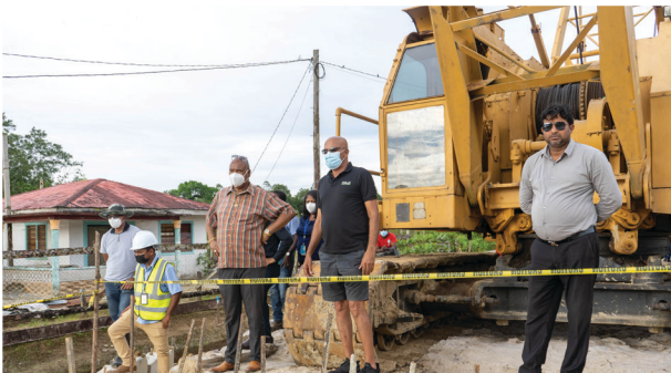
Minister of Public Works, Bishop Juan Edghill MP inspecting a road project in Region Ten
