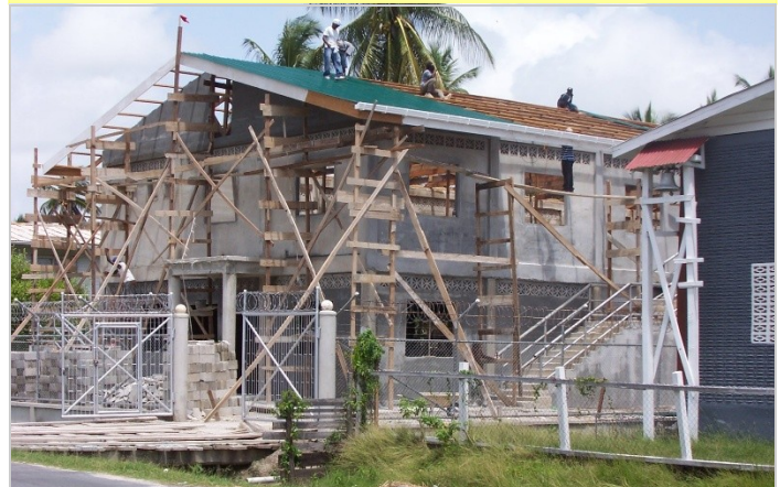
Picture of Tipperary Building construction taken on May 29, 2011
