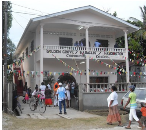
The spanking new multi- purpose community centre at Golden Grove, East Coast Demerara.
